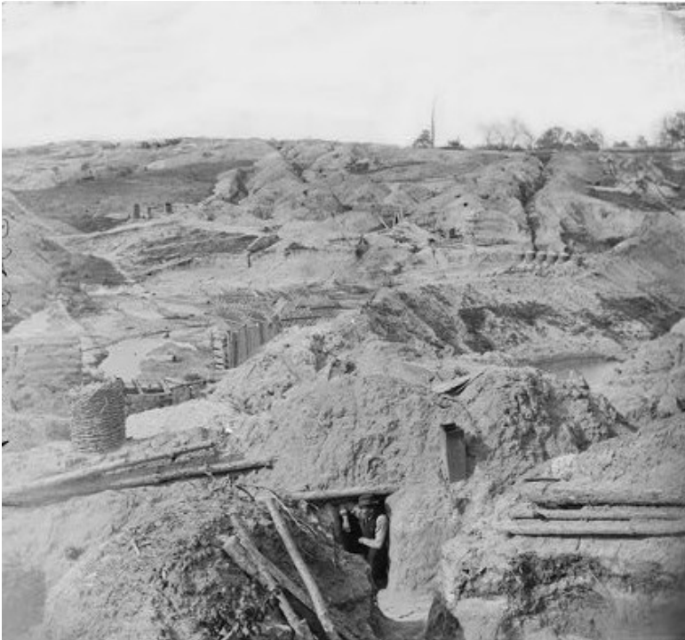
Confederate Earthworks in progress
